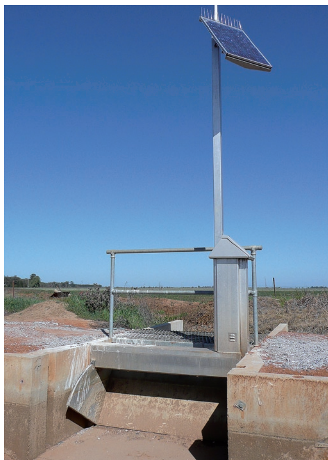
Figure 1. A FlumeGate™, which is an integrated gate and control structure designed specifically for regulating and measuring flows of water on to farm.
