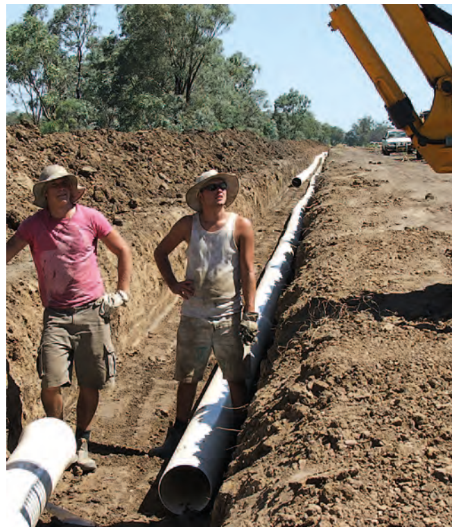
The Estens' development includes a 10.5 km pipeline to pipe bore water to the orchard, which will significantly reduce transmission losses on the lighter soils.
